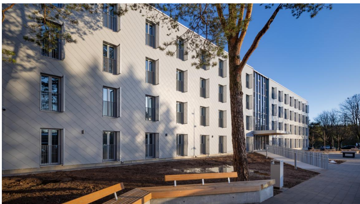
Dormitory of Rakvere Vocational School (photo: Tiit Veermäe).
