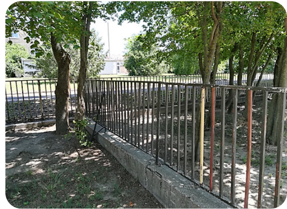
Uncrossable fence. Some fences may only be 1,3 metres high, but are still uncrossable.
