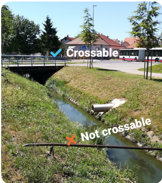
Tubes across the canals are not mapped and shall not be used for crossing!
